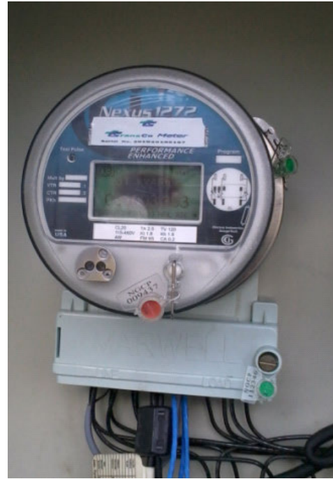
SBMA – Blackened meter display
