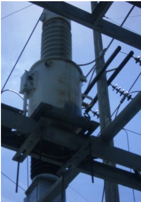
MEPZA 1 – (1) PT Phase B has oil leak; and (2) oil deposit at surface caused by Phase B oil leak
