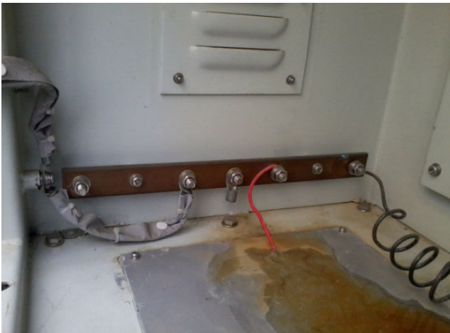
Hanjin – (1) With grounding window for common ground tapping; (2) with space heater to maintain humidity
