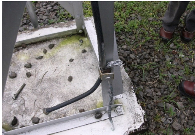
Biñan – (1) Non-standard connection; and (2) poor connection
