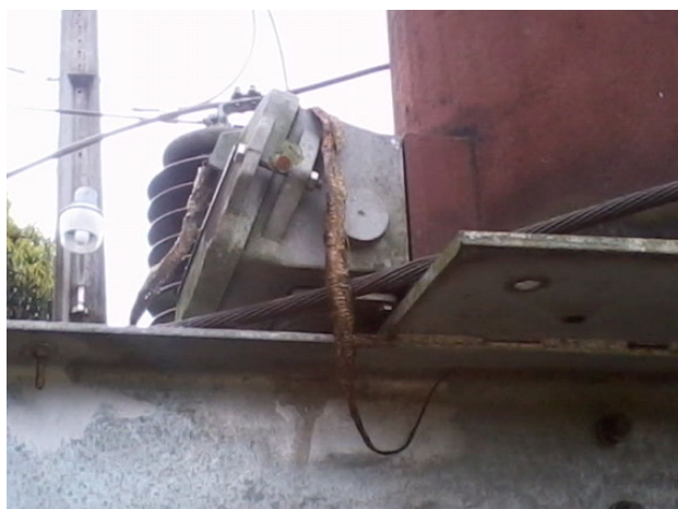
CENECO Alijis – Presence of dead snake on secondary terminal box
