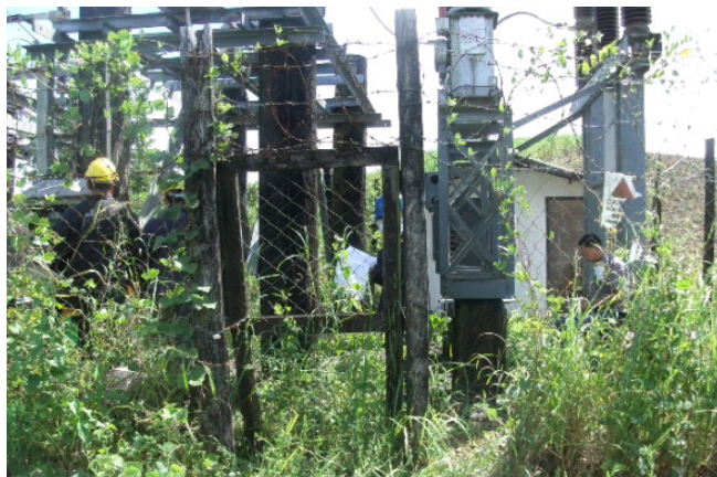
CAPELCO Sigma – (1) Broken perimeter gate; and (2) presence of excessive vegetation
