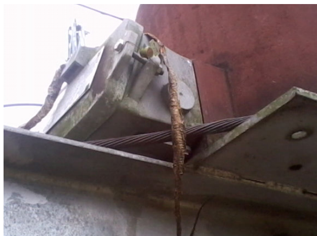
CENECO Alijis – Presence of dead snake on secondary terminal box
