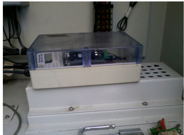
Hanjin – (1) With grounding window for common ground tapping; (2) with space heater to maintain humidity
