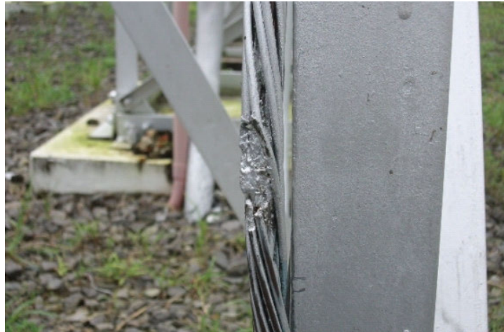
Biñan – (1) Frayed conductor; and (2) melted conductor
