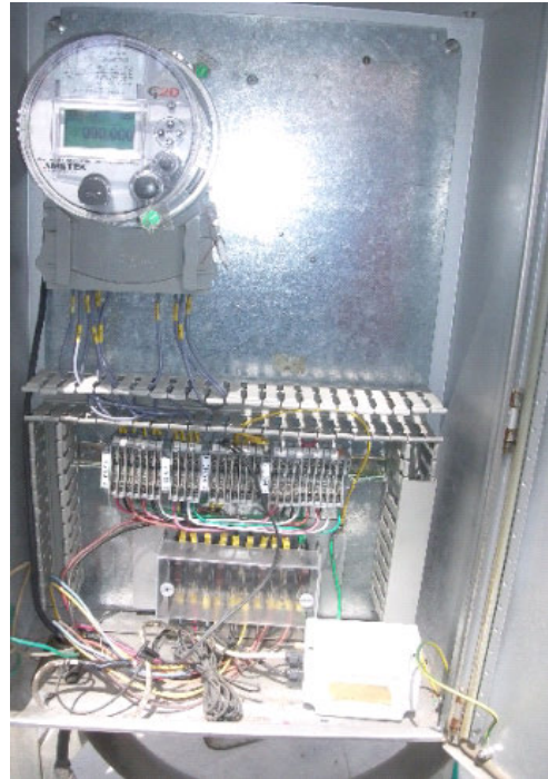
TOLEDO – Ordinary terminal block used
