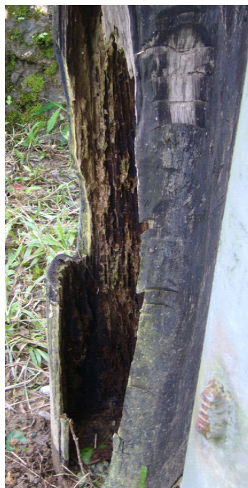
HEDCOR – Rotted Pole Structure
