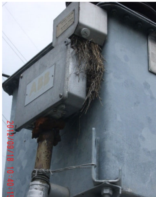
Biñan – Second terminal box with bird's nest
