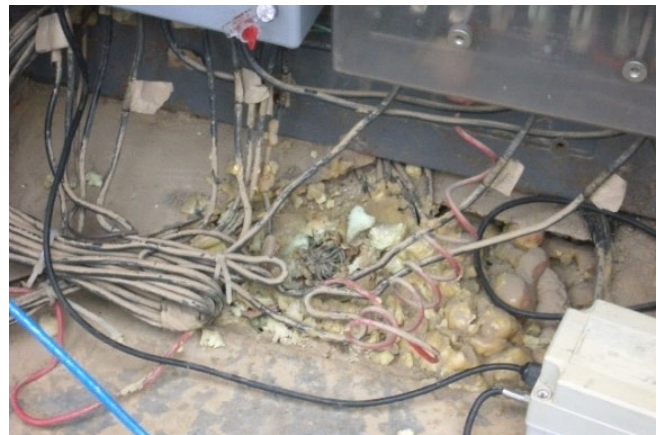
Biñan – (1) Non-standard connection; and (2) poor connection
