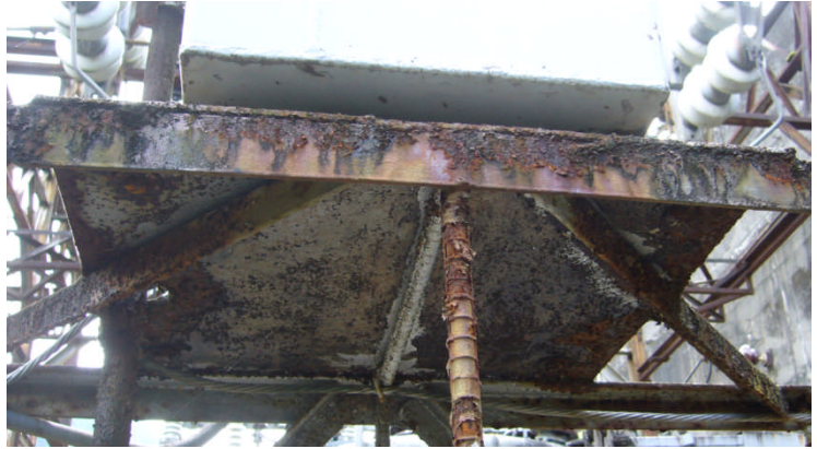
Philex Mining – Rusted facility structures
