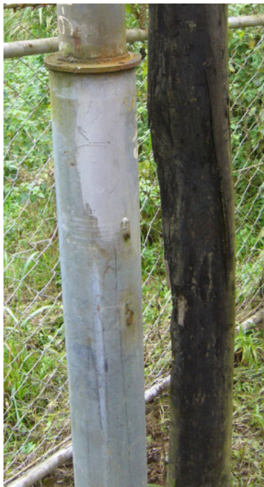
HEDCOR – Rotted Pole Structure
