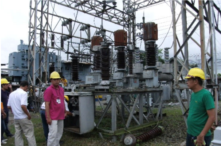
PELCO II Guagua – Low height of structures
