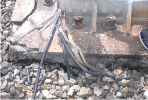
Cebu Thermal – (1) All ground conductors tapped at a single point (structure ground); and (2) ground connection using ordinary solderless connector
