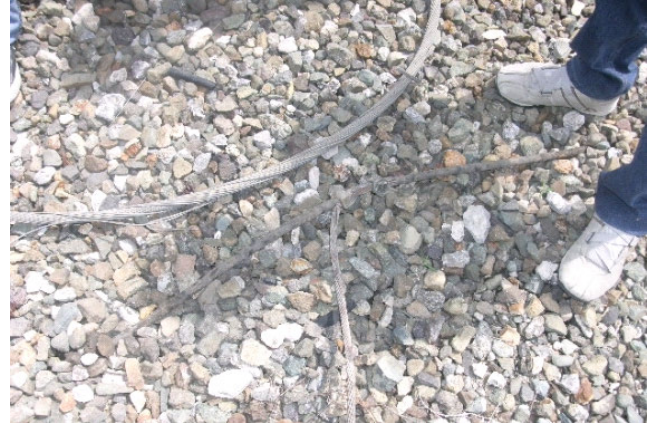
Cebu Thermal – (1) All ground conductors tapped at a single point (structure ground); and (2) ground connection using ordinary solderless connector
